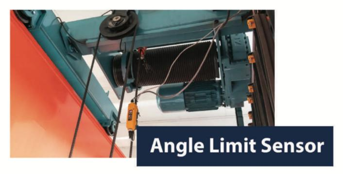
Rope angle limit sensor It is a sensor with 1 relay output to prevent the crane from performing the load lifting function with an angle of more than the adjustable limit value of the rope in two axes to increase the crane and operation safety.
